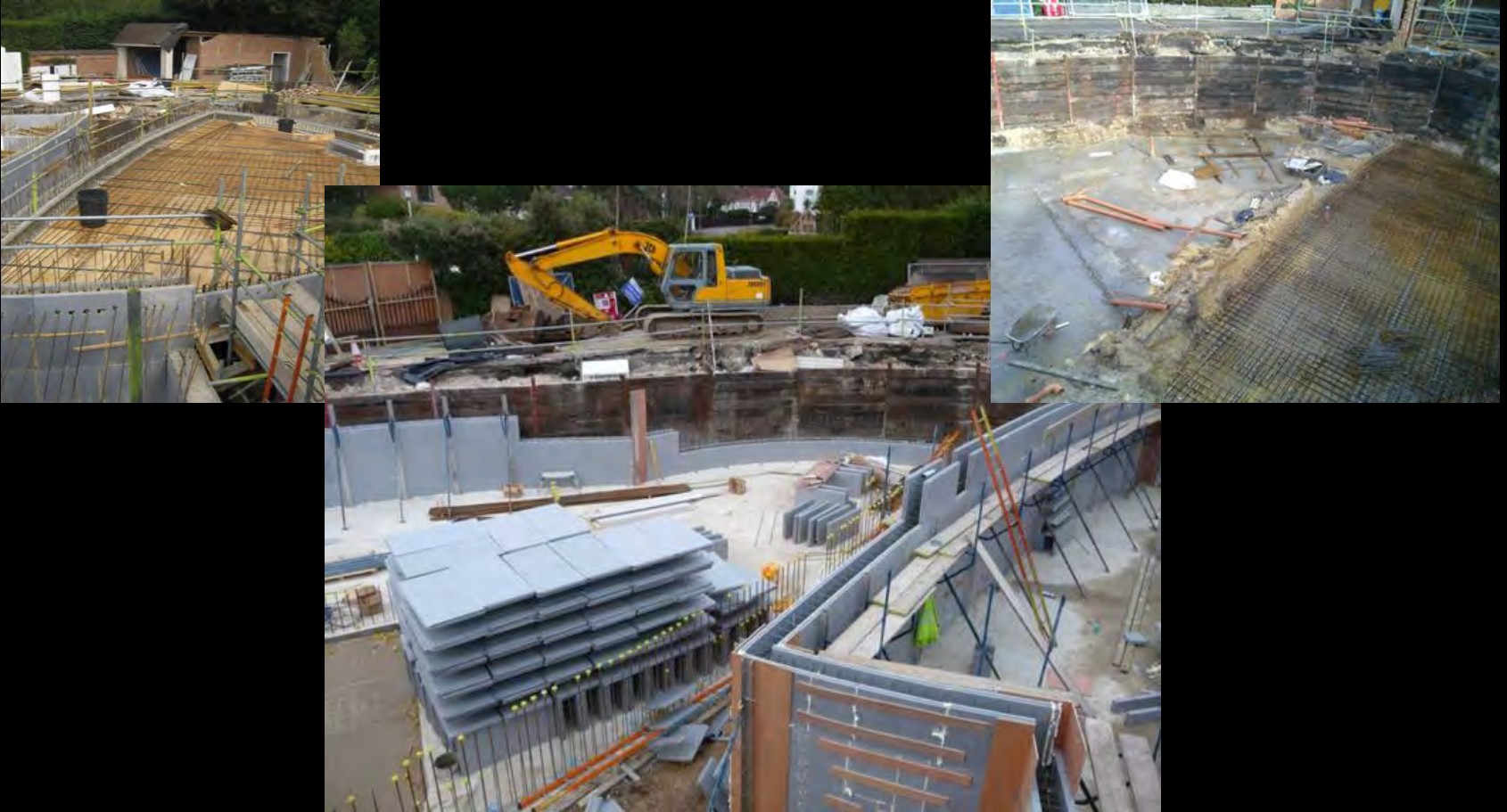
Early construction photos showing the piling, foundations and petal shape forming to the property
