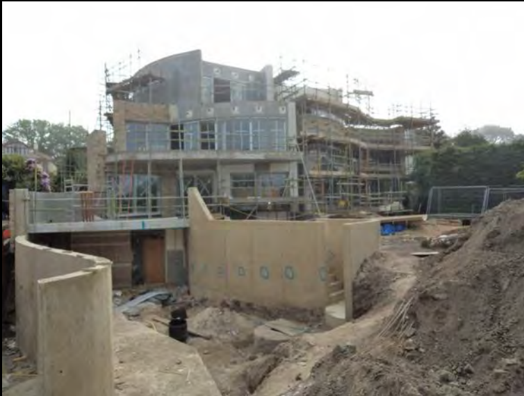
Curved walls to underground garage in formation
