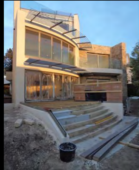
External steps under construction and mineral wall colour render applied to property
